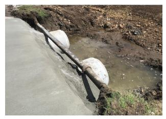
What started as a simple cleanup of the **storm drain at Oronogo and 10**<sup>th</sup> **street** turned into a much larger job than anticipated. Crews discovered that the metal culvert on the east side was decayed beyond repair and had to be completely dug up and replaced. Good thing now is that the area was cleaned out at the same time and we believe we will be able to get mowers in the area that once was impossible to mow.
